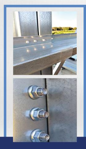
On site COLD FORMED main frame is typically both bolted and screwed together using pre-drilled plates. COLD FORMED buildings can require some cutting/coping and drilling of braces on site.
