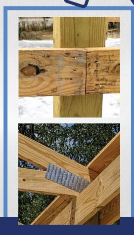
On site a Post Frame buildings main frame is typically connected using steel fastenings and plates. Many connections need to be cut and assembled on site.
