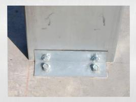
Structural steel buildings bolt to the foundation (slab, piers, strip) typically using cast in anchor bolts which are not supplied with the building kit.
