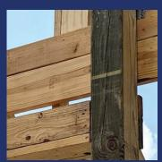
Post Frame type, color, grain, finish (rough/smooth) will vary over a building. Timber moisture content varies. Post Frame has been treated with chemical preservatives to prevent it from decay and insect damage.
