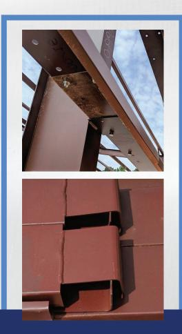
On site a Structural Steel main frame is typically bolted together with plates already welded in place in the factory. Structural Steel buildings can require some welding and drilling on site.
